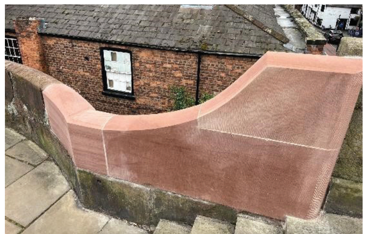
Repairs to Northgate
