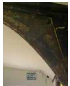
Ordsall Hall restoration work
