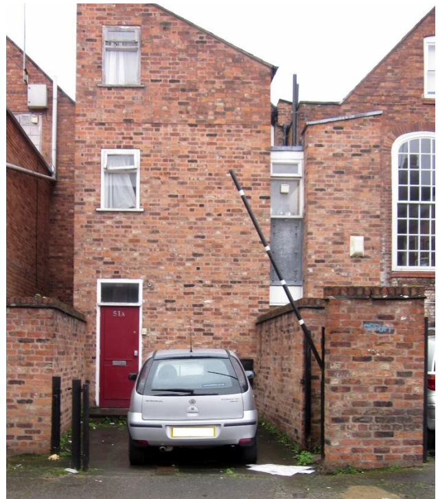
The new external entrance to the flat
