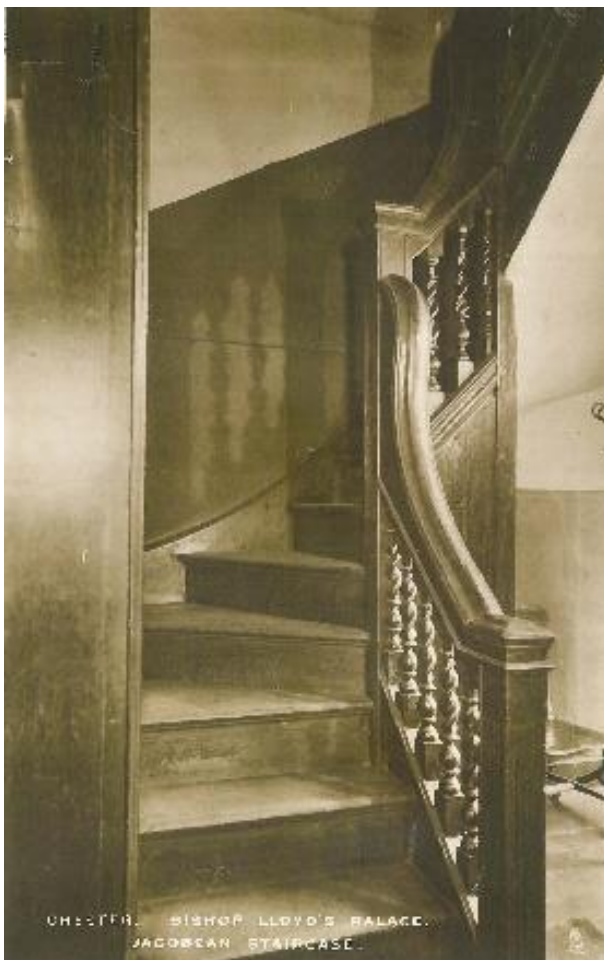
The original staircase to the top floor
