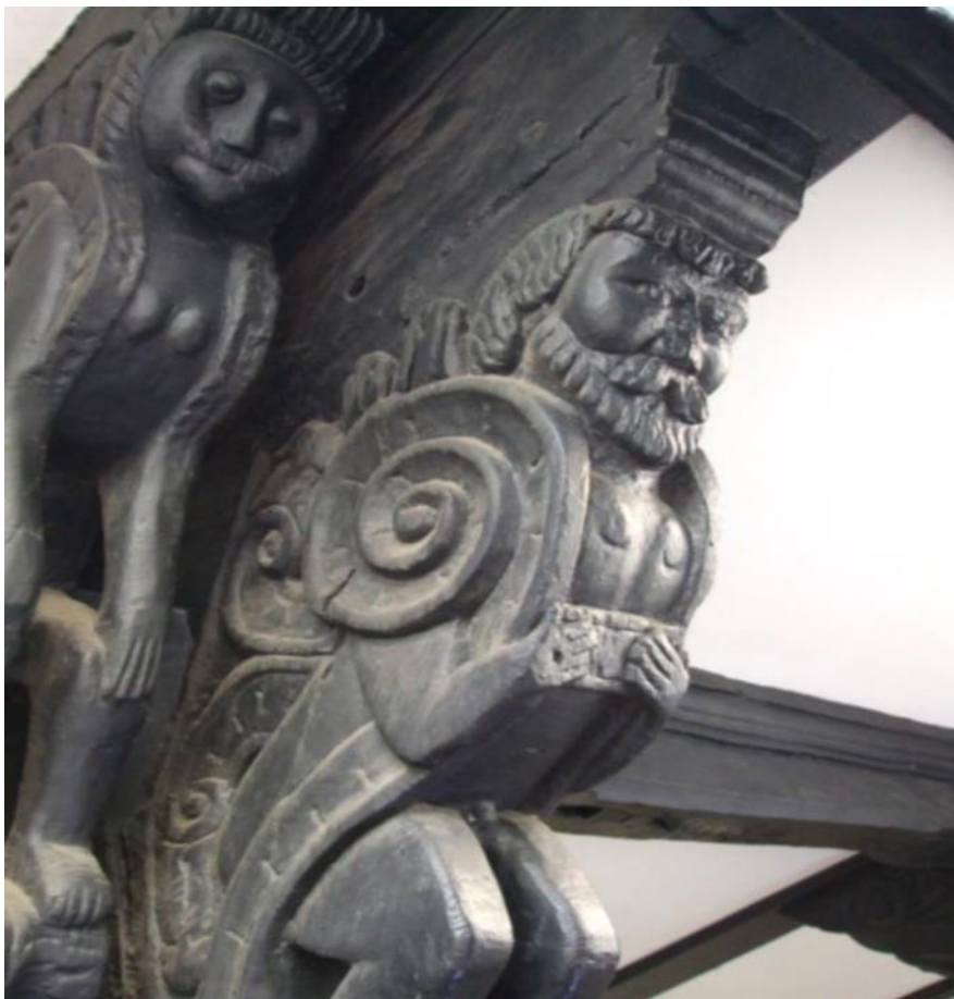
Fig 22: The virile Jacobean giant and its spindlier late Victorian companion. Both, with columns, are supporting the upper part of the building.
