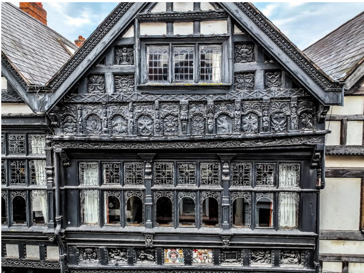
Fig 21: The fenestration in the westerly house. At attic level the original window frame can still be seen. The westerly house has two rows of panes; the easterly house has three rows of panes. The leading is complementary in each house.
