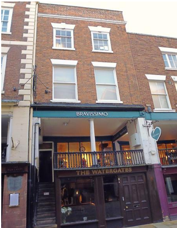
Fig 4: House in Watergate Street. New façade of orange-brown bricks, sash windows and pediment encase the original timber framed building. Done in 1777
