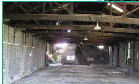
Interior of the Flat Shed
